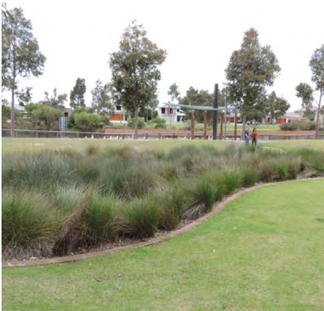
Detention basin planting for storm water filtration
